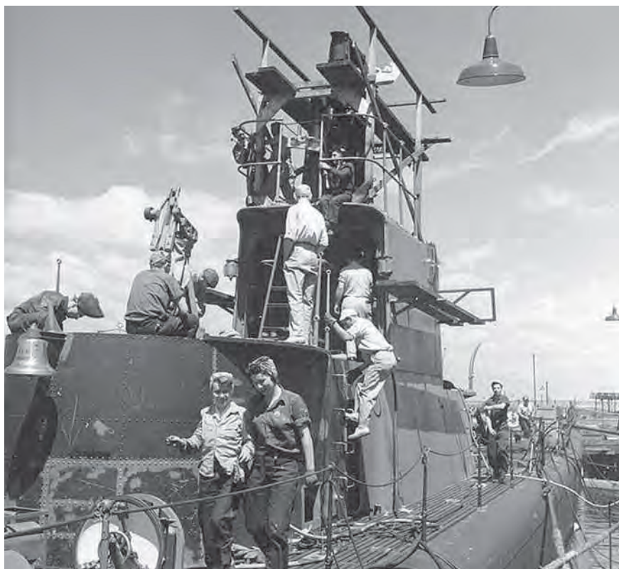
USS Dorado in final stages of construction, August 1943. (Public domain)
